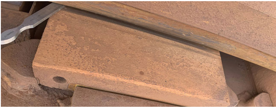
Filler bar beginning to ride up on keeper (at left). Excessive gap also present
