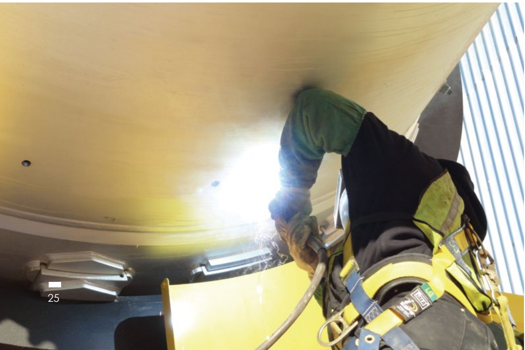
◀ Rotary Drum Repair
