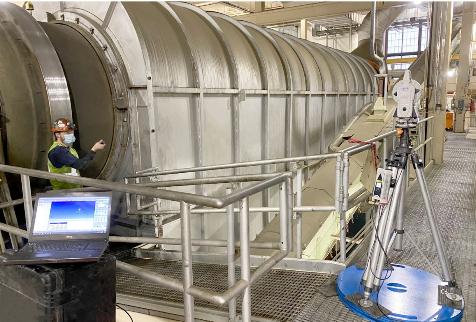
Indirect Kiln Alignment in progress
