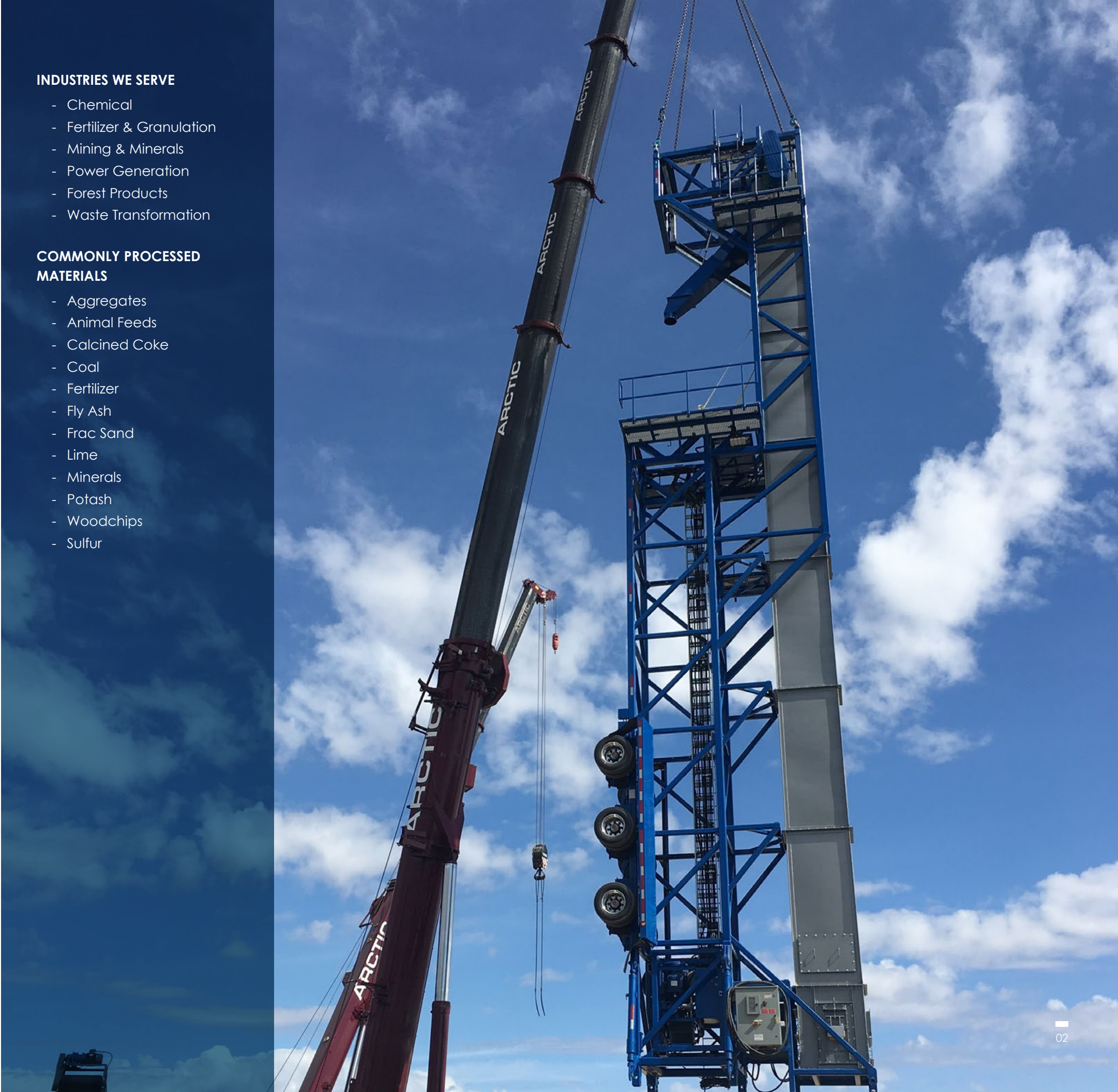
Frac sand unloading/ transfer bucket elevator
