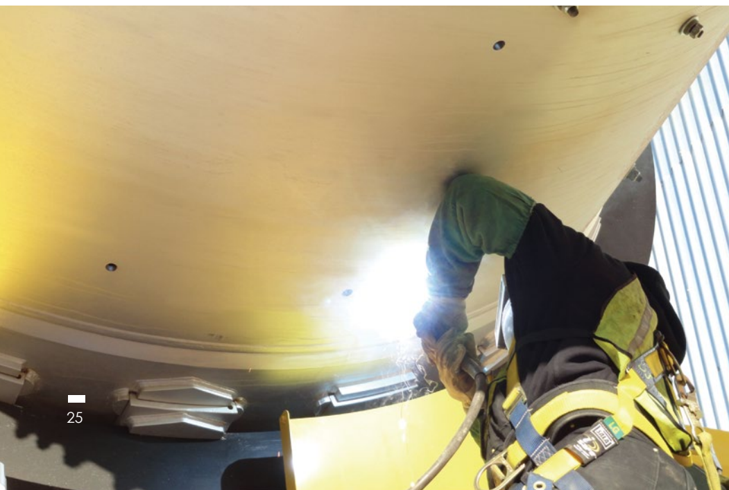
◀ Rotary Drum Repair
