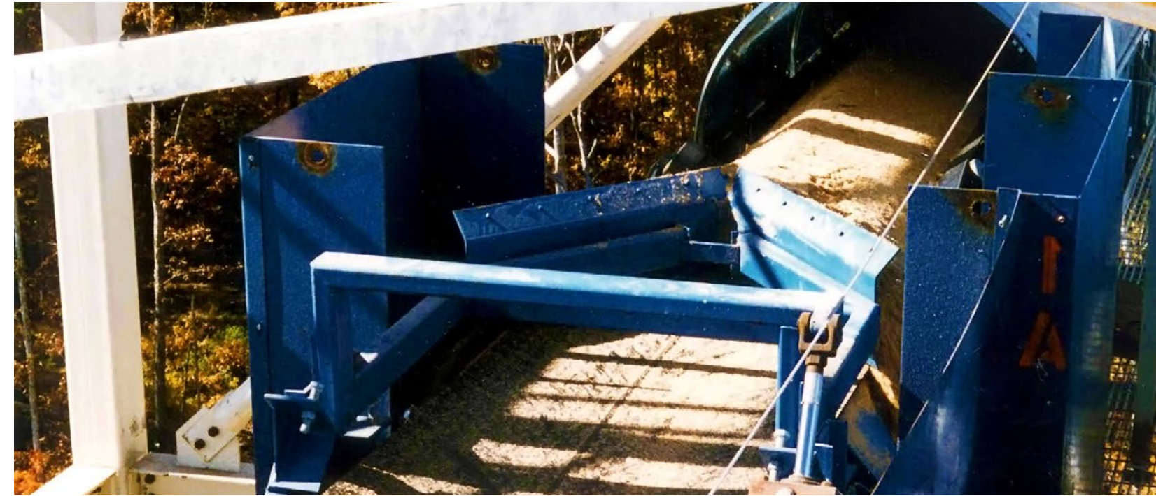
▲ Belt Plow in operation
