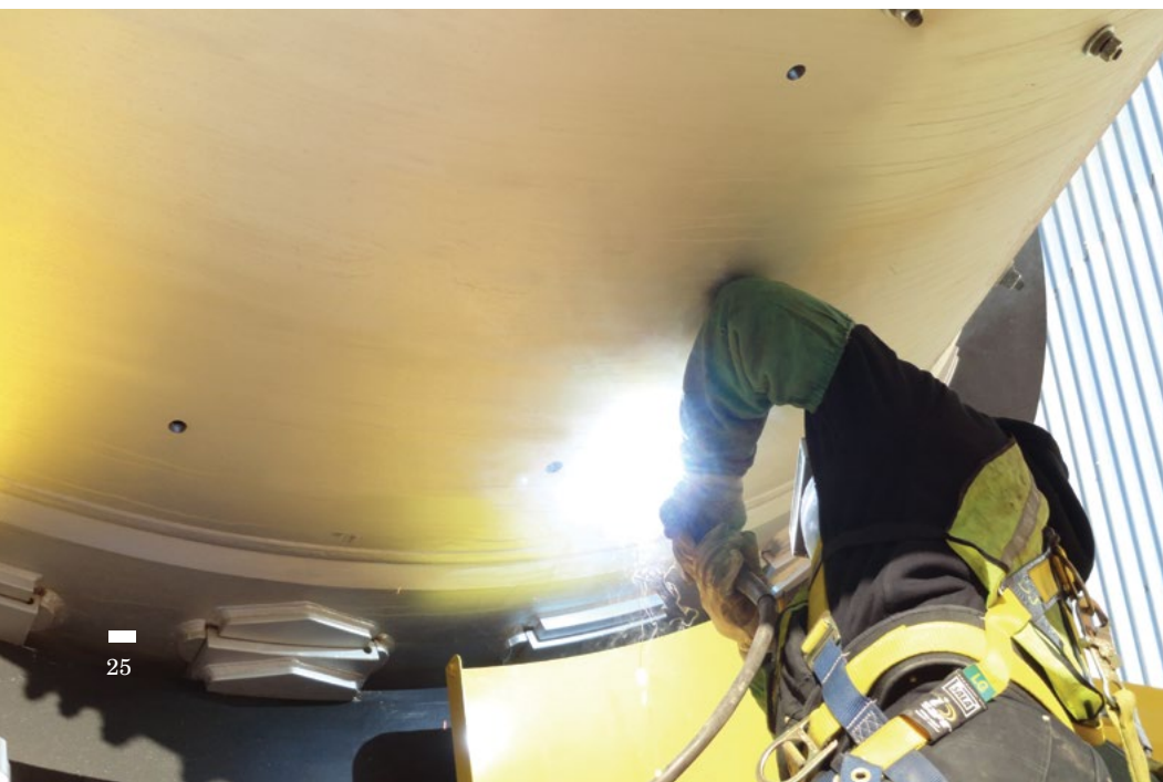
◀ Rotary Drum Repair
