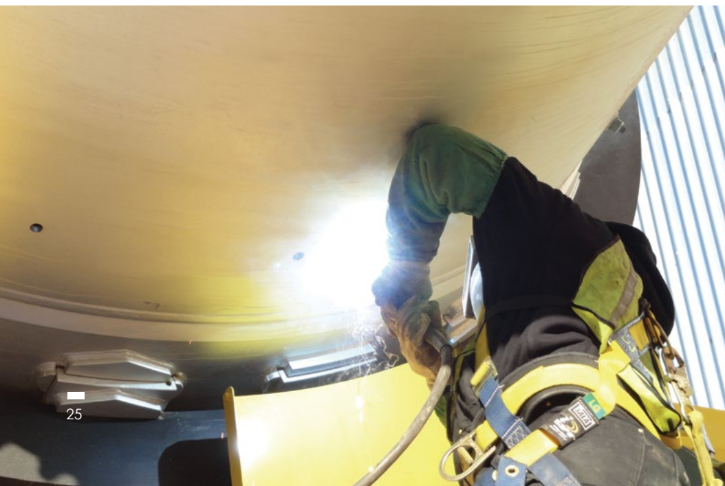
◀ Rotary Drum Repair
