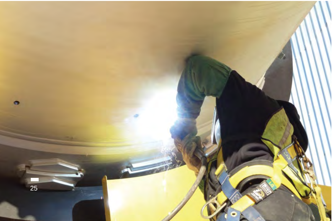
◀ Rotary Drum Repair
