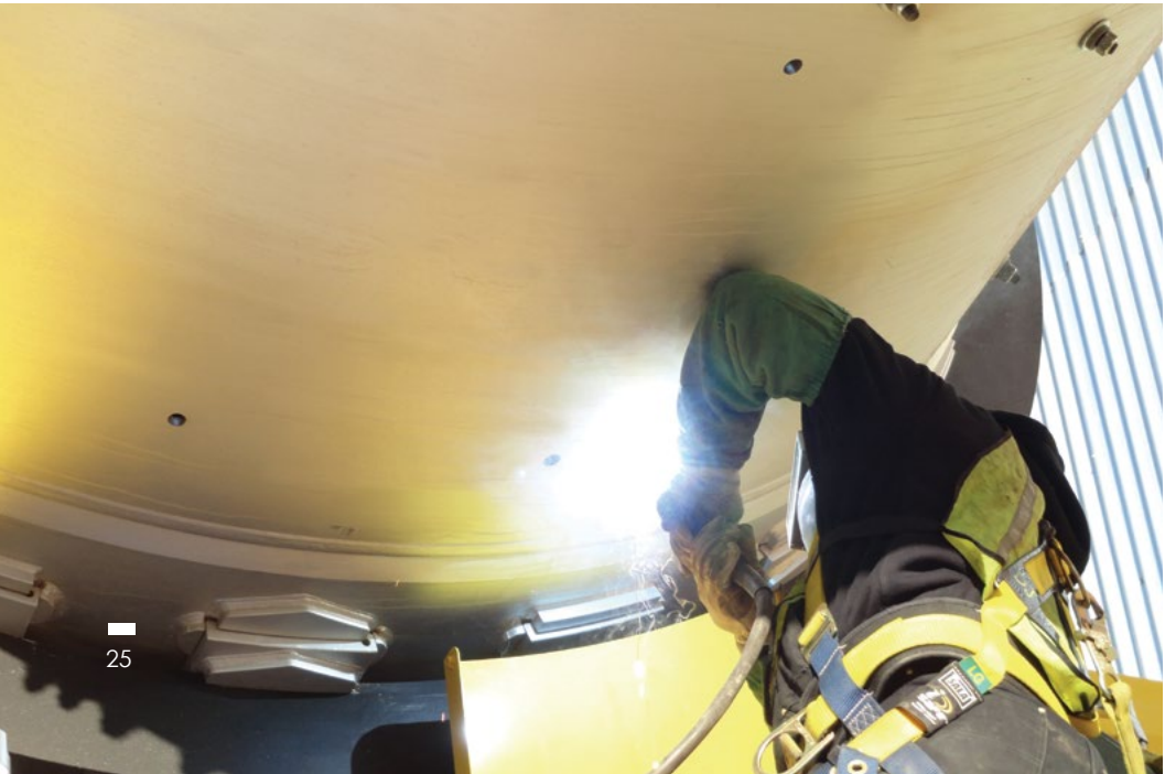
◀ Rotary Drum Repair
